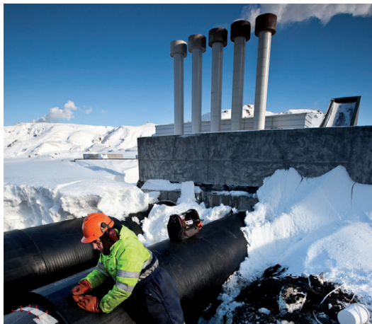
Construction of the Hellisheiðaræð main beside Steam Valve Shed 1
