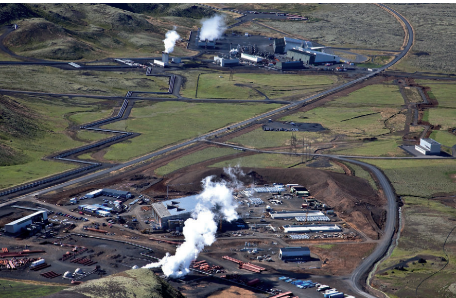
A view of the Hellisheiði power plant construction site
