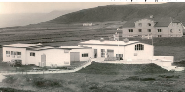
Pumping station and hot water accumulating tank at Reykir in Mosfellsveit
