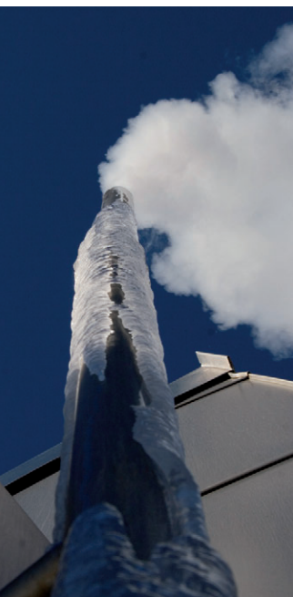
Heating utility installation
