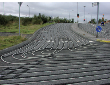
Snow melting system laid into slits made into the tarmac of a Reykjavík street
