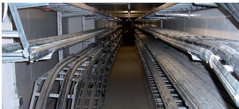
Inside the cable tunnel
