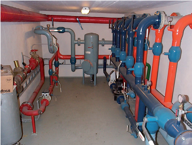
The control centre for snow melting systems serving the Reykjavík city centre
