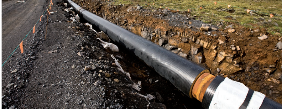
Construction of the Hellisheiðaræð main
